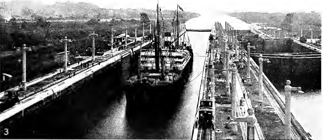
1. Beginning of concrete construction, Gatun Locks, showing cableways for handling concrete. 2. Master wheel and arm for opening and closing gate. 3. Gate beyond vessel is closed, water has reached level of lock in foreground, and vessel is passing through.
