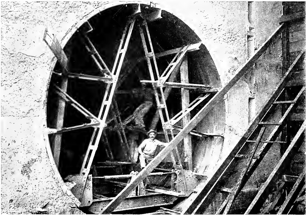
1. Electric towing locomotives passing from one level to the next one above on the lock walls. 2. View showing size of the wall culverts through which the water is let into or out of a lock chamber to lift a ship up or drop it down.
